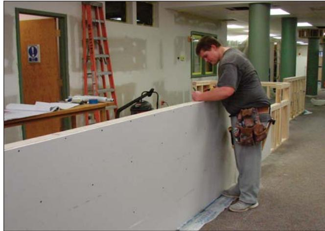
After drywall was installed on the dropped ceiling of the children's stage (left) and the new Circulation Desk (above), it was sanded to get ready for paint.
