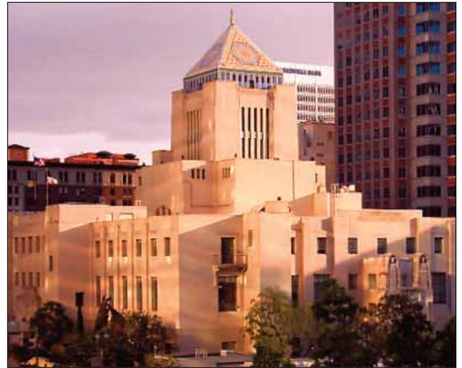
The Central Library was built in 1926 and is a landmark in downtown Los Angeles.
